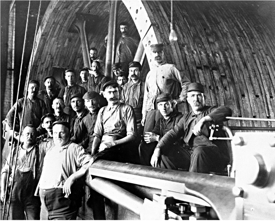
Installation of the great drive wheel, December, 1884. PANB Assorted Photo Acquisitions #5: P61-66.
