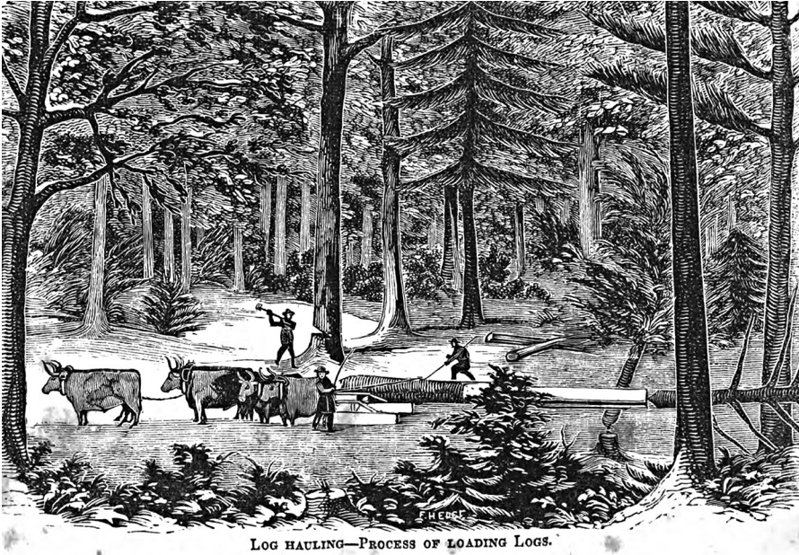
LOG HAULING—PROCESS OF LOADING LOGS.
